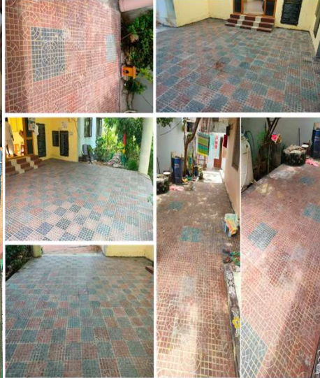
ANTI SKID FLOOR TILES LAID
