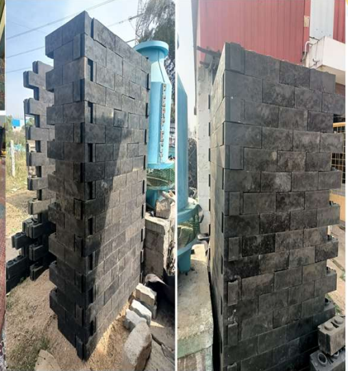
INTERLOCK BRICK CONSTRUCTION
