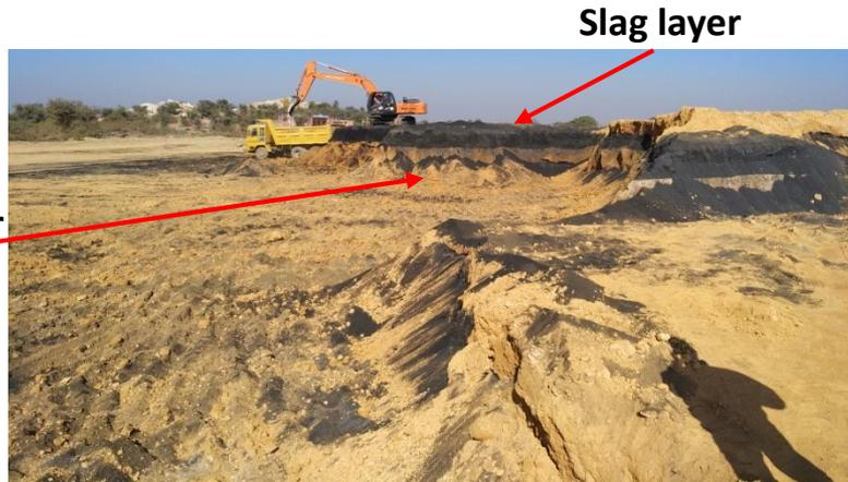
Stacking of jarofix and slag layer by layer
