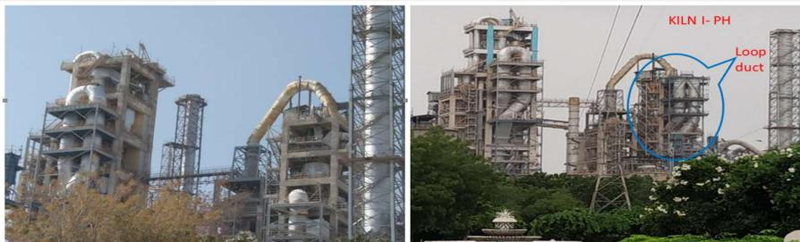
Photographs Showing loop duct modification before and after Birla White
