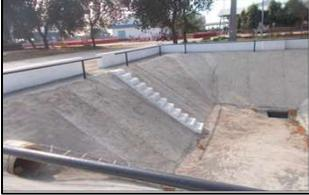
Water reservoir of capacity 380 KL for rooftop rainwater and surface runoff water from parking area
