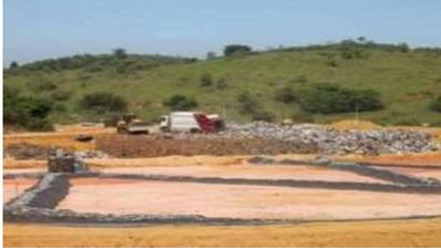
**Landfill Construction:** Geotextiles can also be used for landfill construction projects where it acts as filter fabric on top of waste materials before being covered with dirt or rockfill materials. This helps keep smaller particles from escaping into the environment while still allowing water to flow freely through the waste material layer below so that it does not become saturated and cause instability issues with any overlying soil layers.
